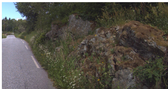
Fto Statens vegevsen
